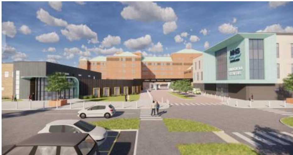
3 - Overall building view
